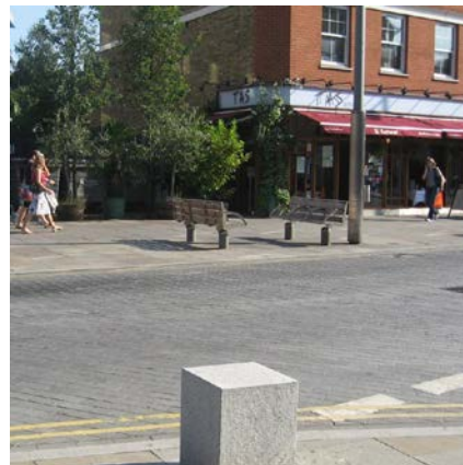
Visual changes combined with road narrowings have reduced traffic speed at The Cut, London
