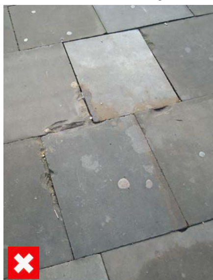
Natural stone damaged when replaced
