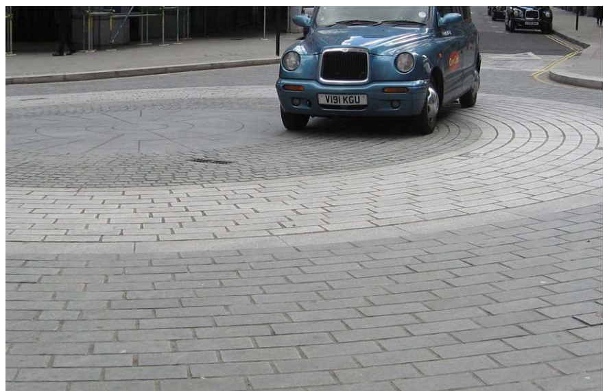
Surface materials at an uncontrolled junction with courtesy crossing help drivers to negotiate
