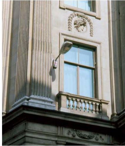
Wall mounted lighting on historic building
