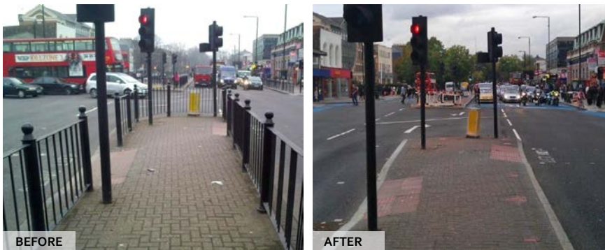
At many of the TfL crossings, guardrailing was removed without any other associated works
