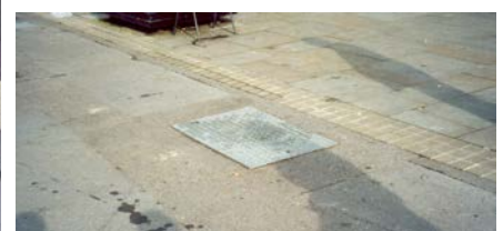
Electricity supply cabinet for street market
