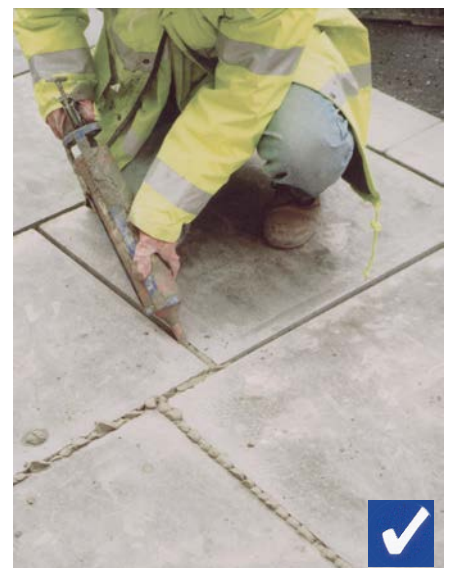
All the slabs should have the same appearance
