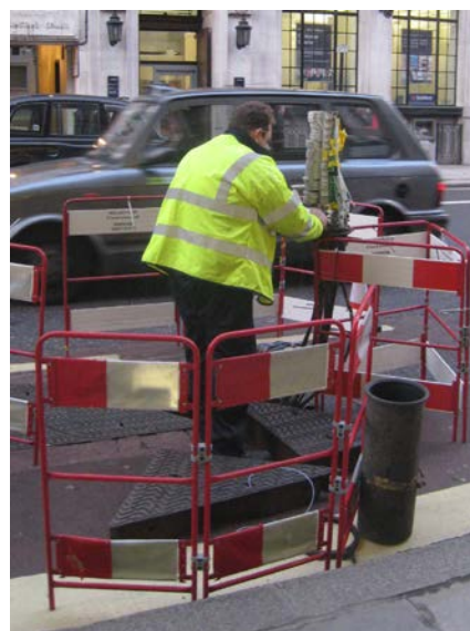
Underground telephone cable cabinet
