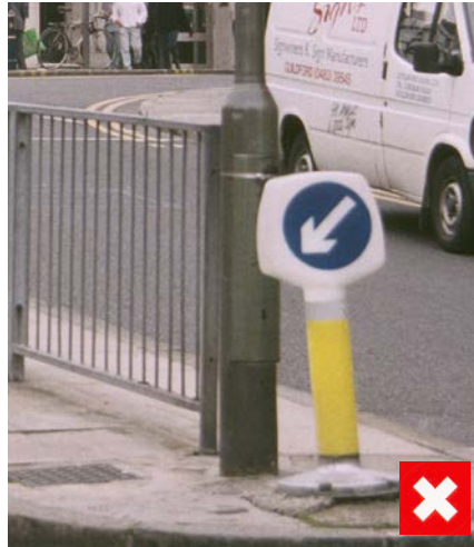
Unnecessary sign and guardrailing
