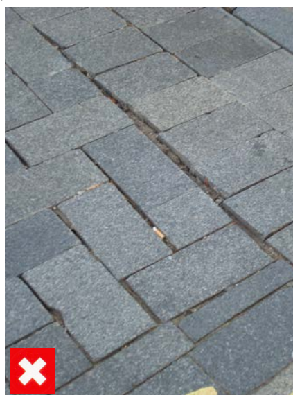
Granite blocks on an insufficiently strong base
