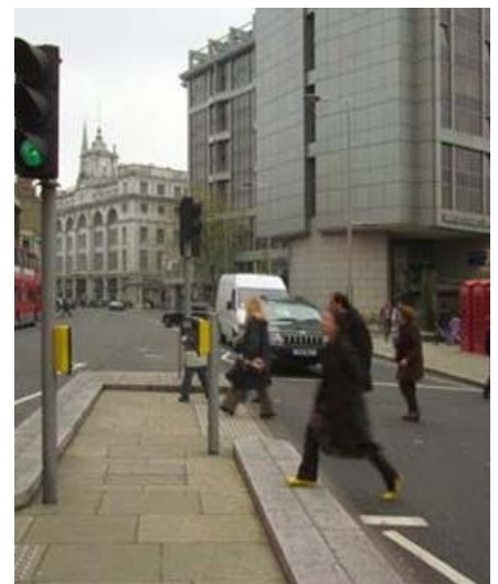
Pelican crossing without guardrailling
