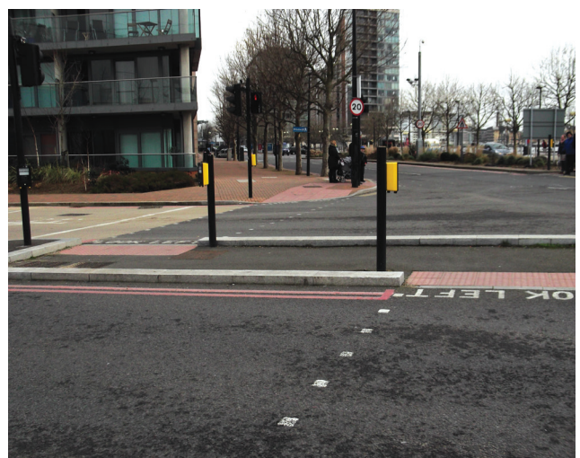
Western Gateway, Docklands: PedX crossing without guardrail
