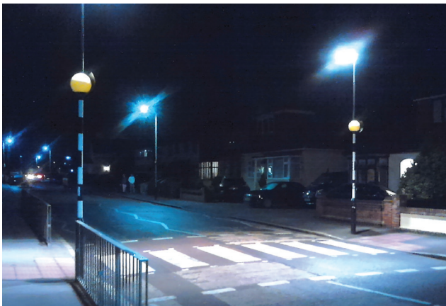
Zebra crossing pedestrian lighting
