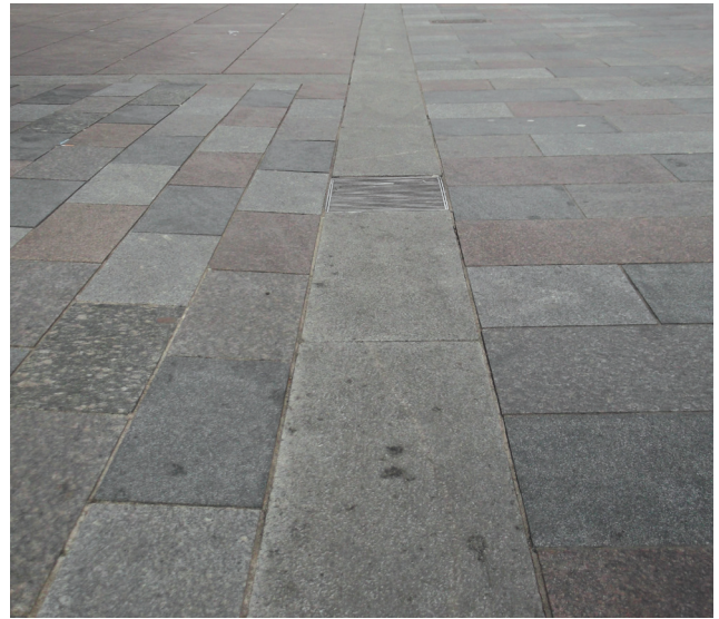
Gentle gradients and a flush channel block leading to pedestrian-friendly gully grating
