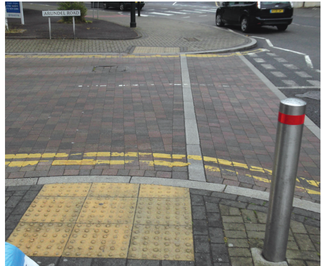
Side road entry treatment using a speed table
