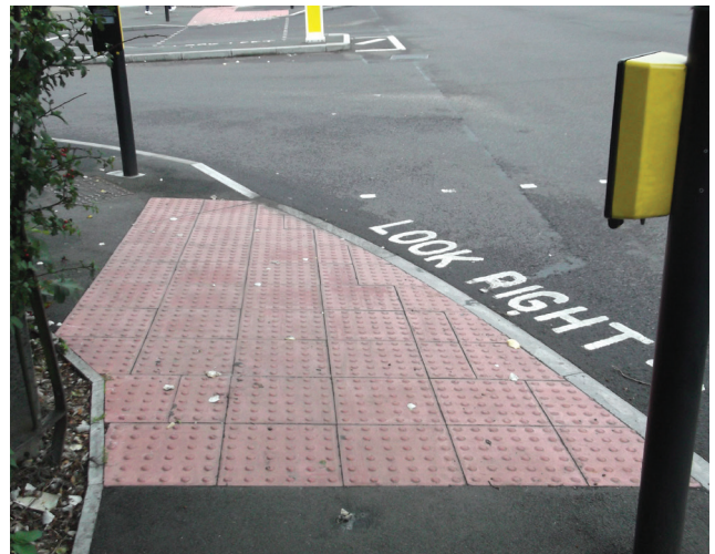
Tactile paving laid in a way that could confuse people into walking across the road at an unintended location road
