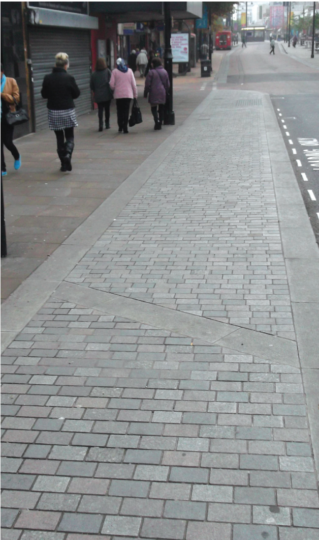
Level surface footway loading bay allows for essential servicing of shops but is fully available to pedestrians when loading is not taking place
