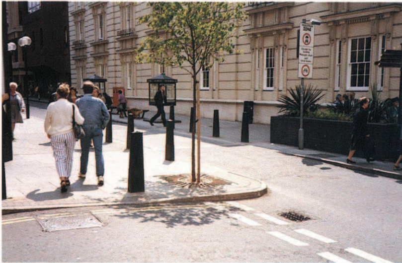
35: Widened footway in Queen Street has improved the area for pedestrians. The flat top hump at footway level assists pedestrians when crossing and the street furniture and planting help define the route traffic has to take. (Photo: Devon County Council)
